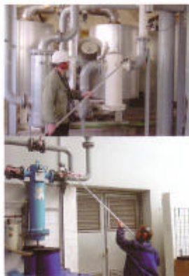
Picture above: Leak detection by an air sound detector
